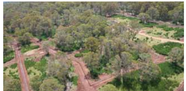
Aerial photo of Devil Ark just prior to completion of construction phase 1
